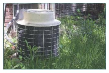
around the unit should be trimmed back at least 2 feet (0.6 meters) to allow for adequate airflow around the condenser.
